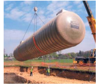
Water Tank installation
